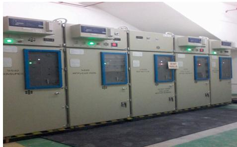
Figure 3. Installation of the magnetic actuator driven switchgear in the trial site
