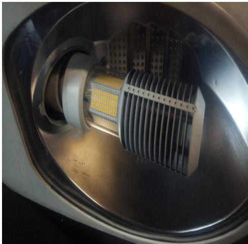
Figure 4. LED lamp in 150W HPSV light fixture
